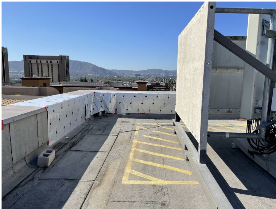
Figure 3: PIM Foil deployed on parapet wall in front of site antennas
