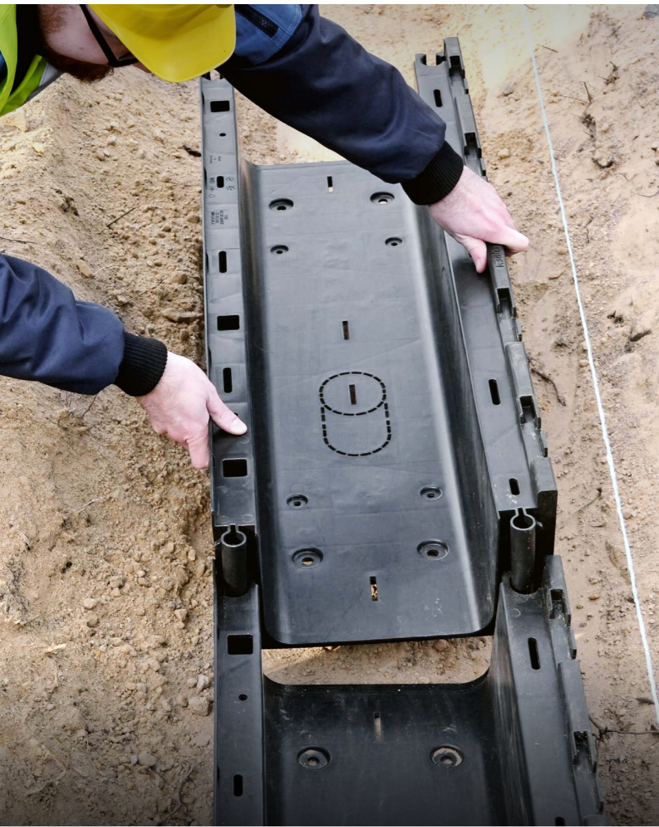
Fig. 1: Connecting of the cable ducts
